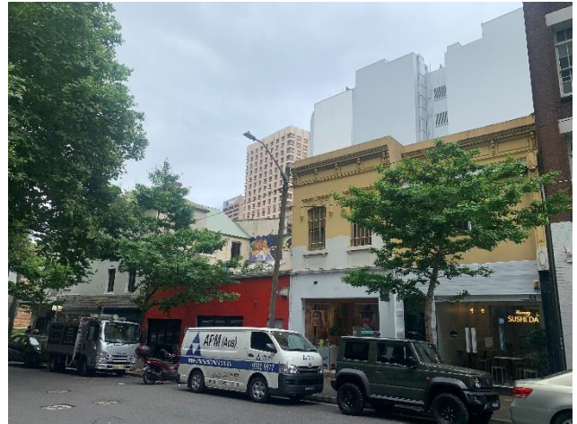
Figure 6 – View of secondary façades on Reservoir Street
