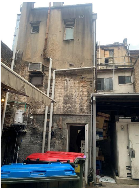
Figure 21 – Rear dock/service yard accessible via Foster Lane.
