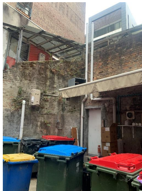
Figure 22 – Rear dock/service yard accessible via Foster Lane.
