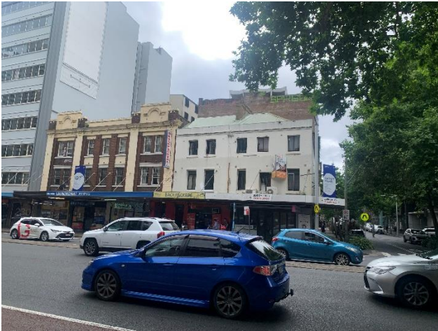
Figure 5 – View of primary façade on Elizabeth Street
